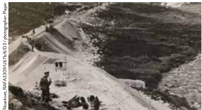
Fillings for the polar railroad on Saltfjellet.
