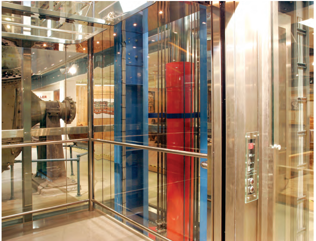
Right: Hydraulic ram as seen through the lift car
